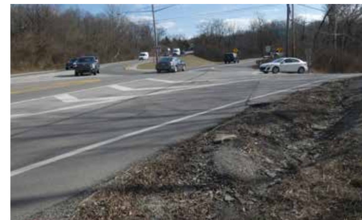
Ohio 32 looking east to Eight Mile Road
