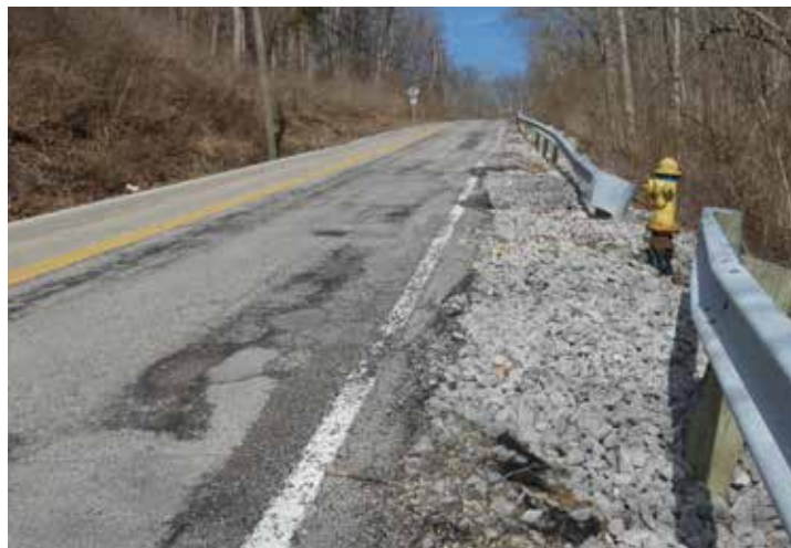
Asbury Road upgrades include repaving and repair of the degrading roadside.
