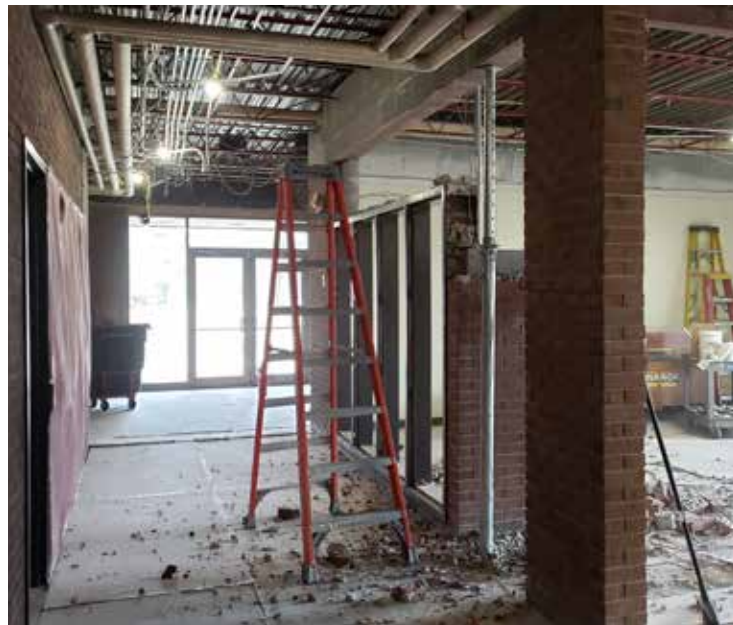
Renovation of the Anderson Parks Recplex includes many upgrades including handicap accessibility.
